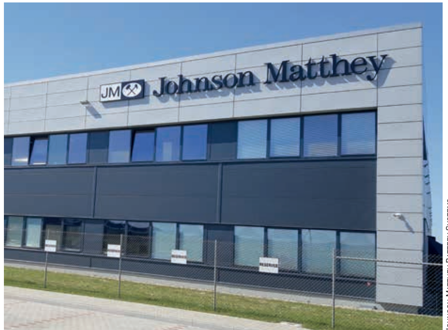
JOHNSON MATTHEY BATTERY SYSTEMS
